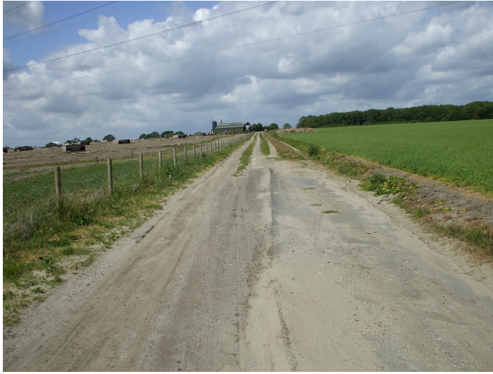
SU 0295-5634 looking north-west.
